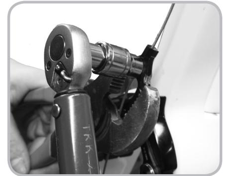
Figure 10.6. Tightening the cable clamp nut
